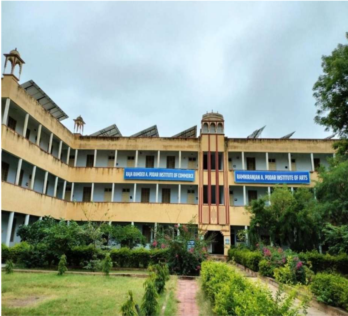
New Building – Arts & Commerce Block
