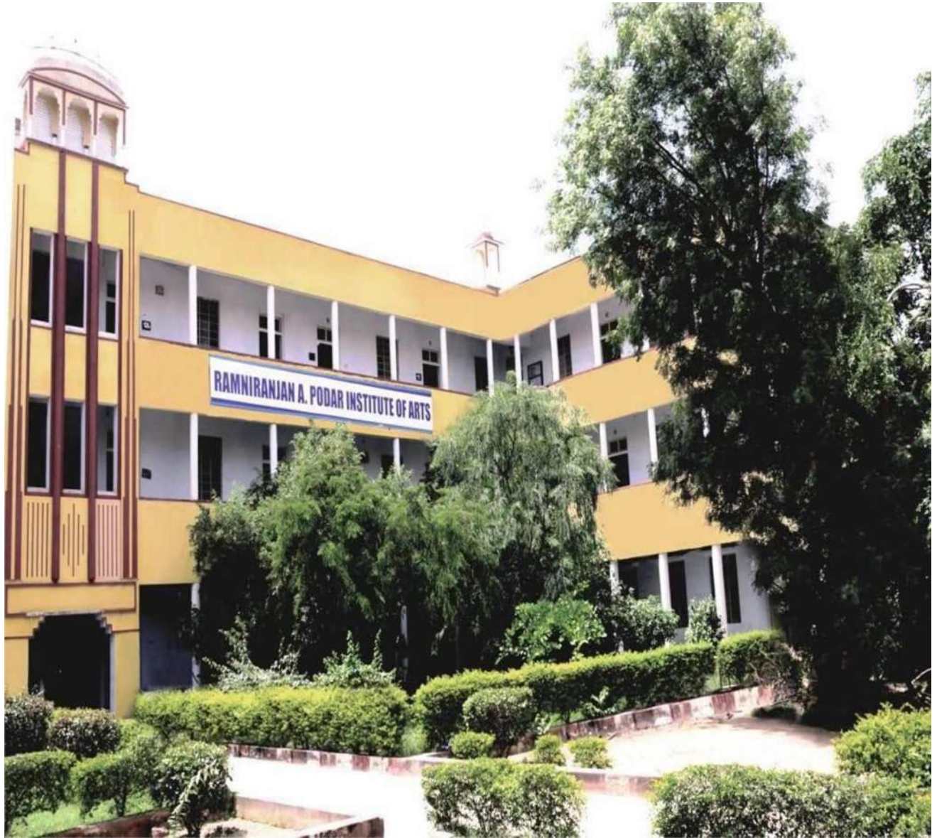
New Building – Arts & Commerce Block
