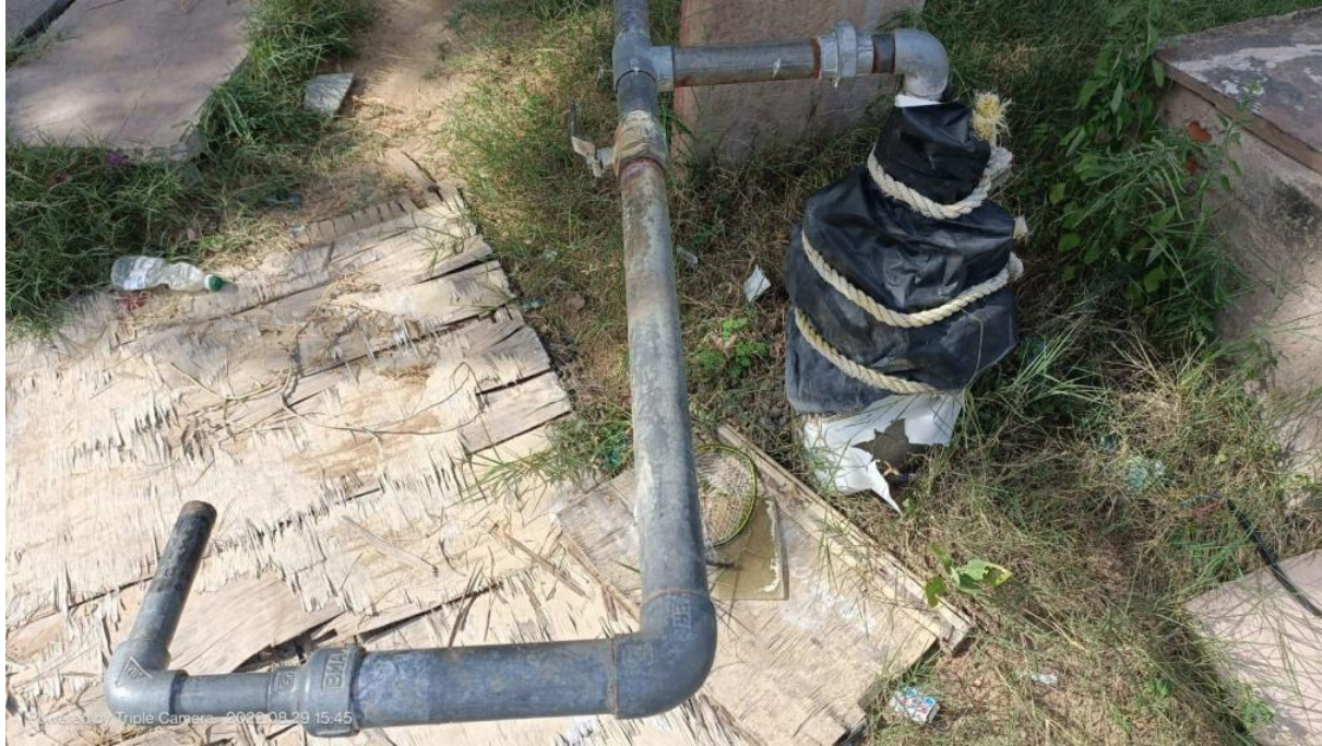
Bore well point in Main ground
