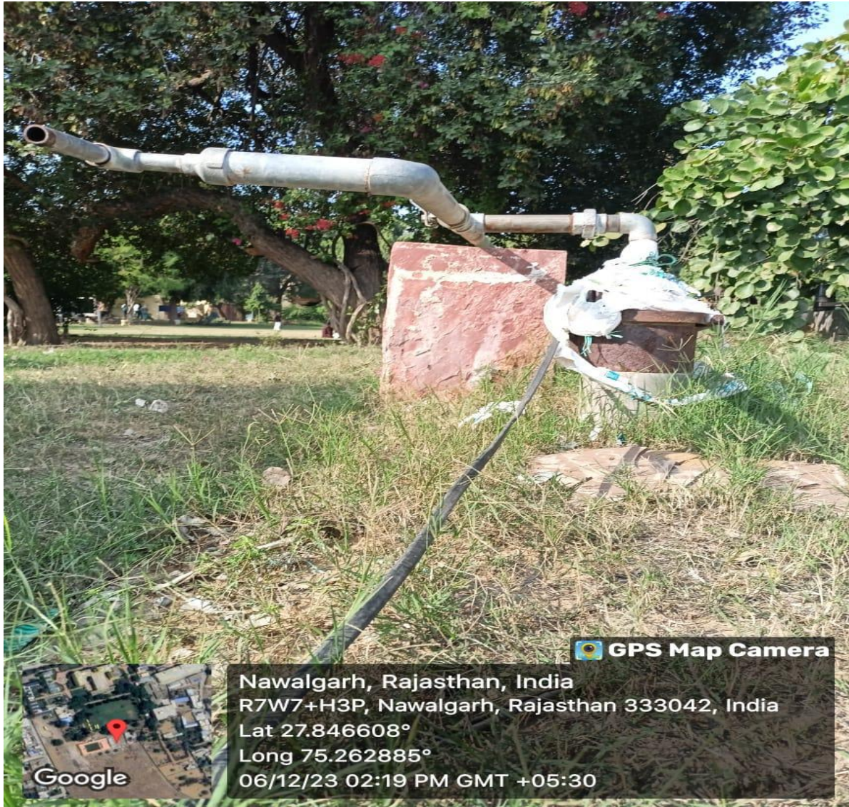
Bore well point in Main ground
