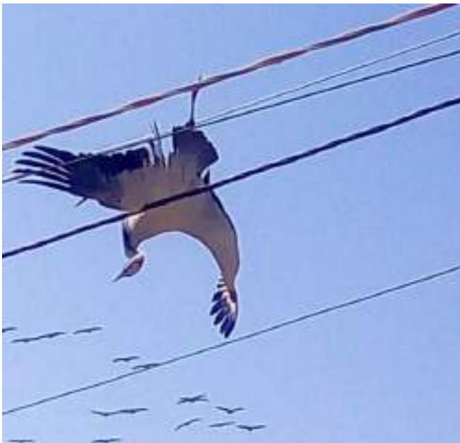
Fig -7: Demoiselle crane collapsed with electric wires.
