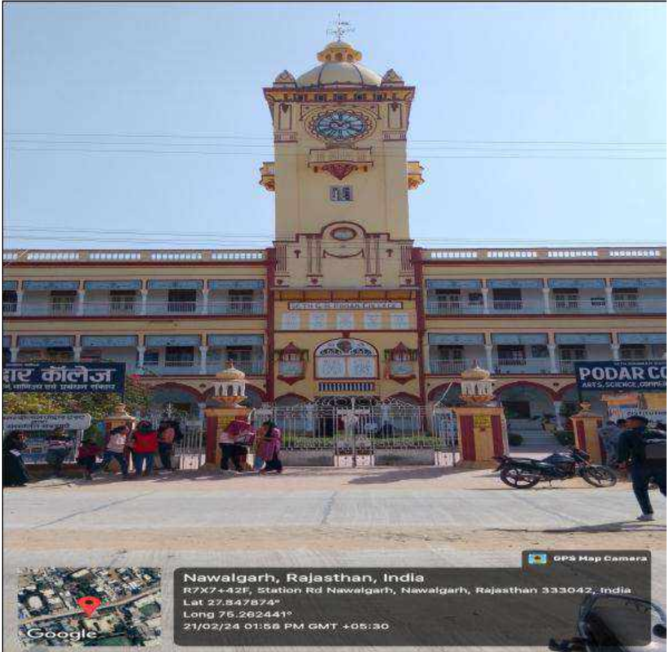
Front view of Science Block in Main Building of College
