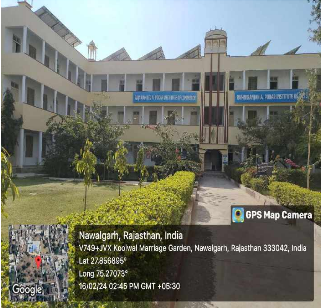
New Building – Arts & Commerce Block
