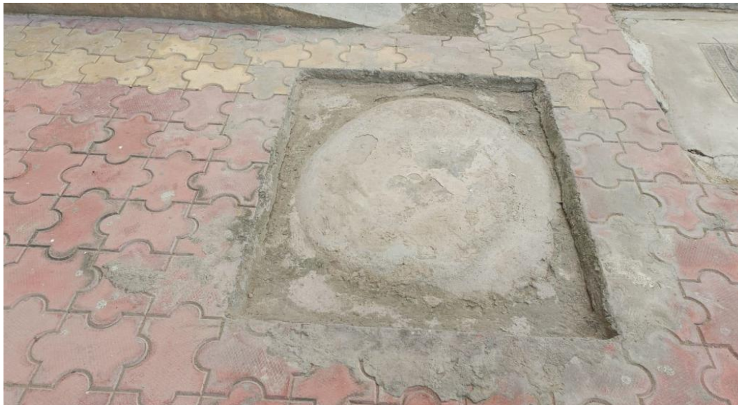
Safety Tank of Toilets
