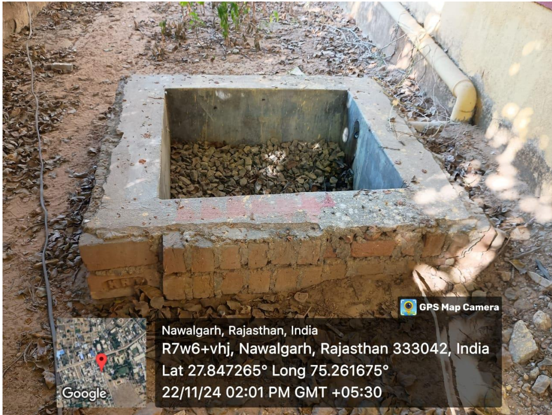
Water Harvesting System: Construction of Underground Tank
