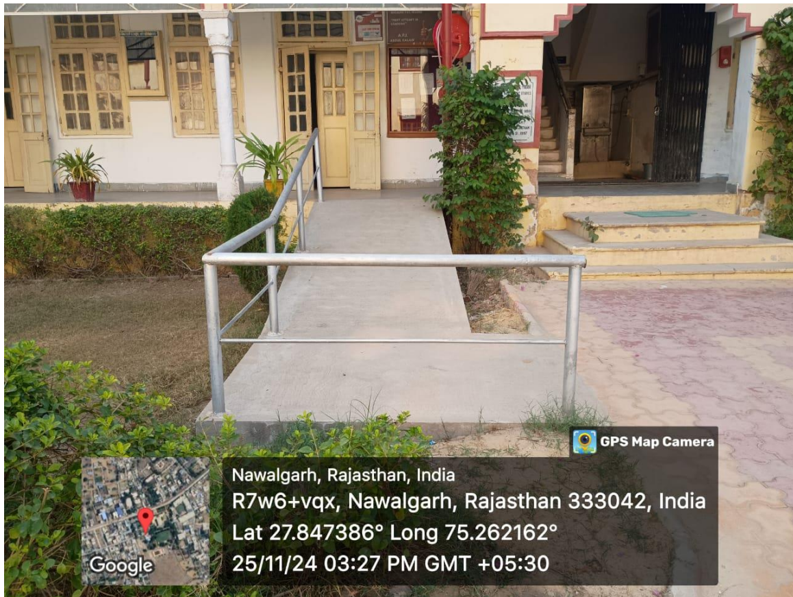
Ramp at Academic Block
